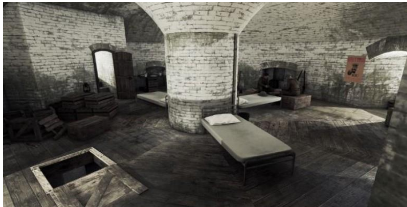
View of the first floor, showing the "mushroom" supporting the gun platform and the trapdoor leading to the ground floor.
